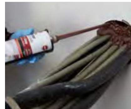
Fill pipe and cable spaces: 3M™ Fire Barrier Rated Foam Pg 87
